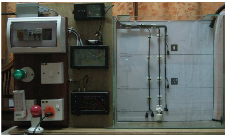
Fig. 1: Flood detection system
